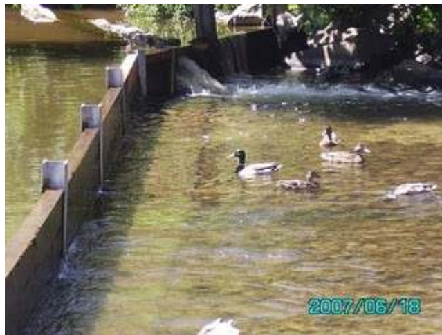
Plate 3. D River Dam installed. Fish passage maintained.
