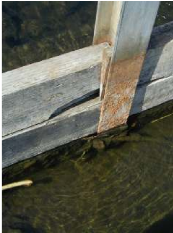
Plate 2. Boards secured in dam with wedges.
