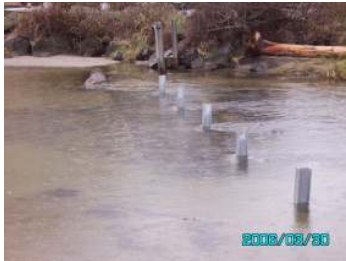
Plate 1. Dam at D River. Stanchions only.
